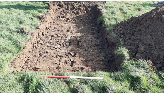
Plate 5: XC211 TP02. Looking south-east. Scale 1m
