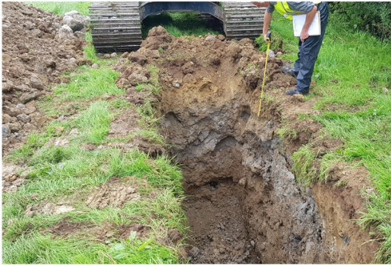
Plate 1: XC201 TP01. Looking north-east
