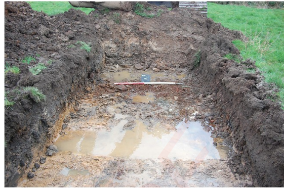
Plate 8: XC215 TP03. Looking south-east. Scale 1m
